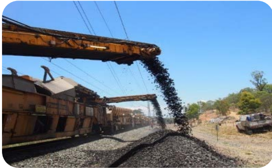
Ballast Undercutting Machine in Operation
