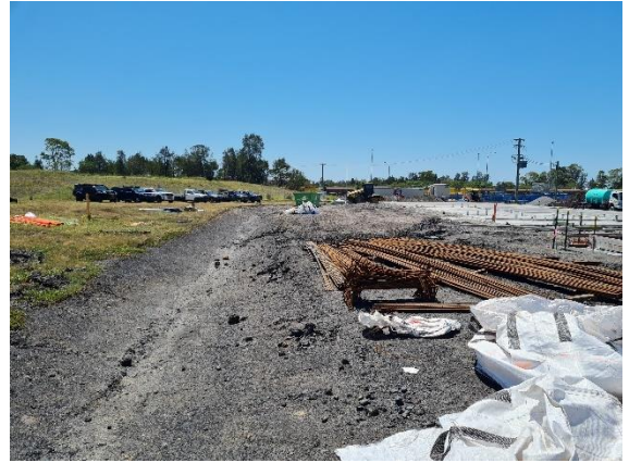
Figure 2: Existing drainage line bordering site (March 2023)
