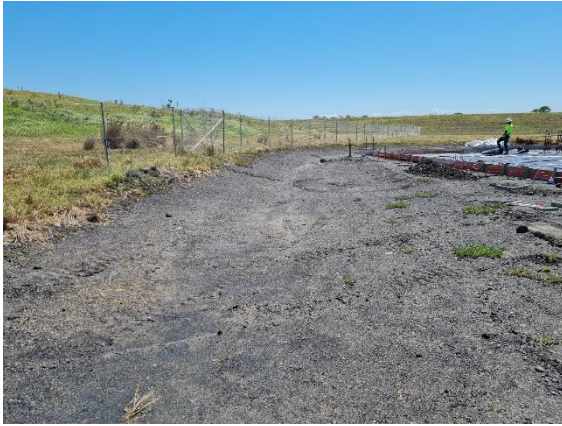
Figure 1: Existing drainage line bordering site (March 2023)
