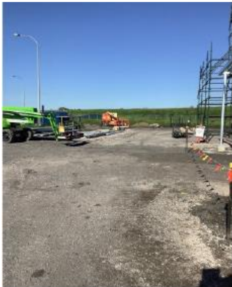
Figure 5: Onsite shed area (April 2023)
