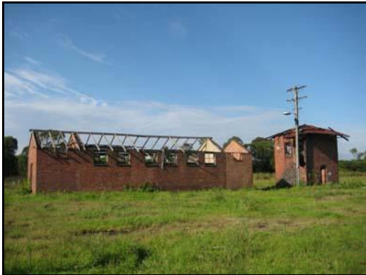
Figure 29. Bath-house and Control Cabin
