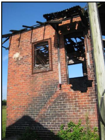
Figure 31. Control Cabin. EJE Heritage
