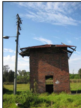
Figure 32. Control Cabin. EJE Heritage
