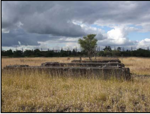
Figure 37. Conveyor Belt Support Footings . EJE Heritage
