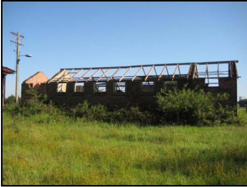
Figure 33. Bath House. EJE Heritage
