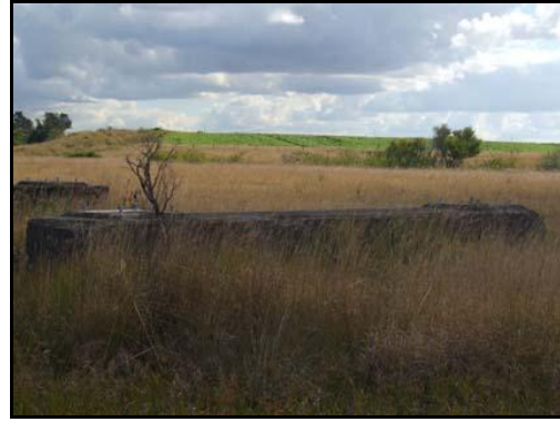
Figure 38. Conveyor Belt Support Footings. EJE Heritage
