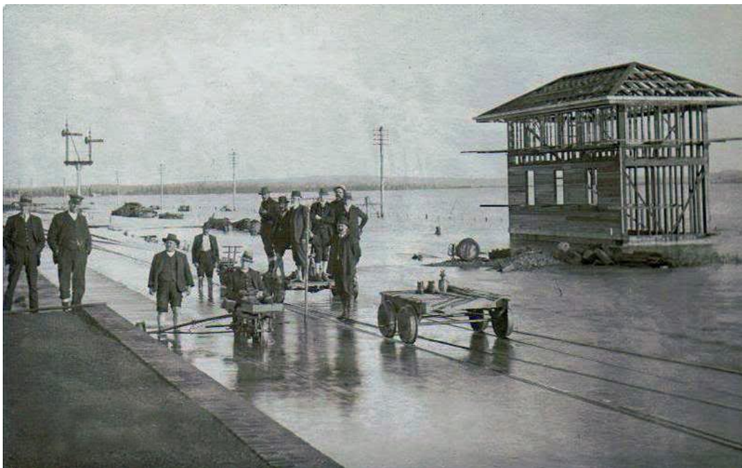
Figure 9. A photograph taken from the eastern end of the first Hexham station. The new signal box is half completed, but point rodding and the interlocking machine (signal box levers) have not yet been installed. The island station platform is visible. The later site of the Coal Preparation Plant is behind the investigating party. Late Mrs Rita Cameron
