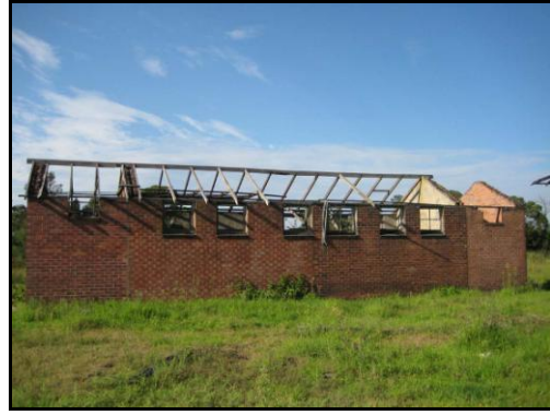
Figure 34. Bath House. EJE Heritage
