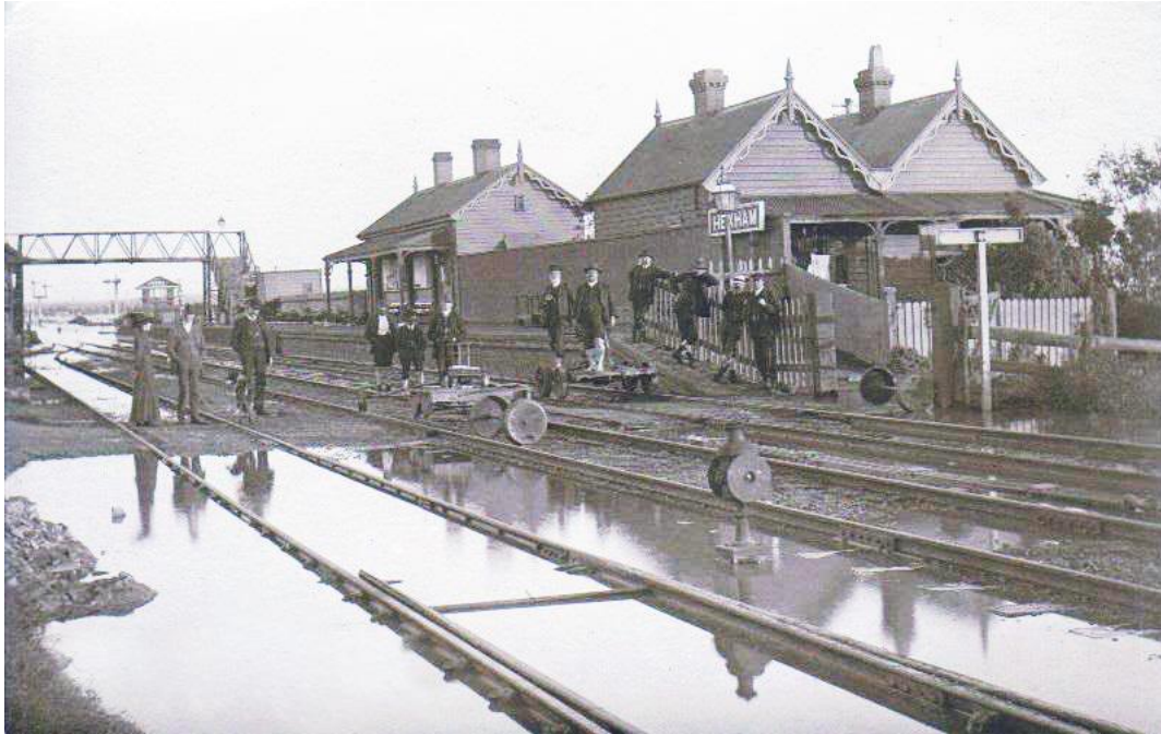
Figure 8. Hexham station, Station Master's residence and signal box before their demolition for the Coal Roads project. The photograph may have been taken in May 1913, when flooding is known to have occurred; running lines are being investigated for damage or obstructions. The new Hexham signal box is seen beneath the footbridge. Late Mrs Rita Cameron
