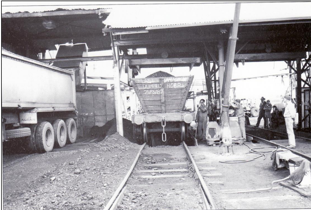
Figure 28. Last coal wagon to be dumped at the coal preparation plant 21 September 1987. Brian Andrews, Coal, Railways and Mines
