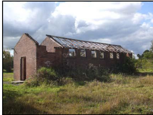
Figure 36. Bath House. EJE Heritage
