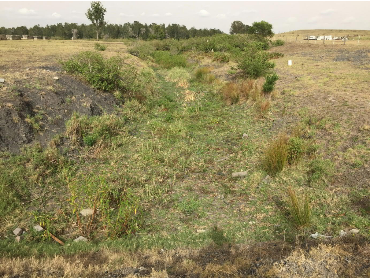
Plate 2. Photo showing a stormwater drain towards the northern end of the proposal footprint.
