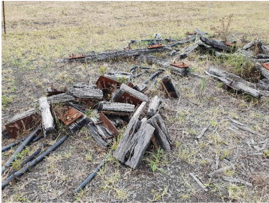
Figure 5.5: Presence of timber and metal pieces within the study area (Source: Jacobs, 2019)
